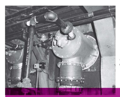
These Low NOx ATP Burners are firing a new hot strip mill reheat furnace.
